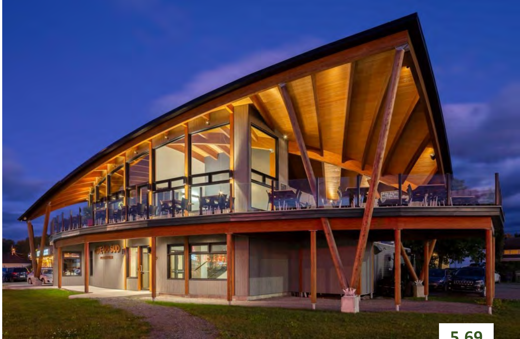
Cross Laminated Timber Construction at a Brew Pub in Quebec, Canada
