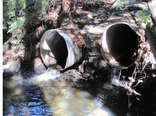
Lyon Creek Culvert – NE 195 th St. – Barrier to Fish Passage and Structurally Deficient
