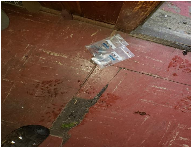
Photo #11: Samples 11720-70,71/71QA: 9"x9" Red VFT on black mastic (on wood.) (5% Chrysotile, <1% Chrysotile) Location: Building 6 Living Room
