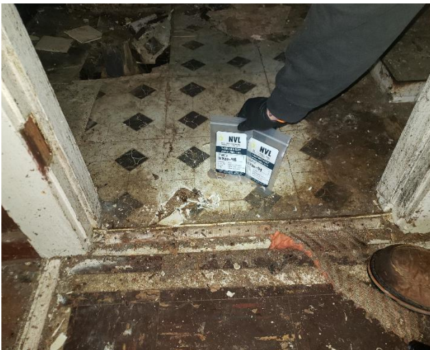
Photo #7: Samples 11720-48 & 49: 12"x12" White and black VFT on brown mastic (on wood) (46% Chrysotile) Location: Building 9 Bathroom
