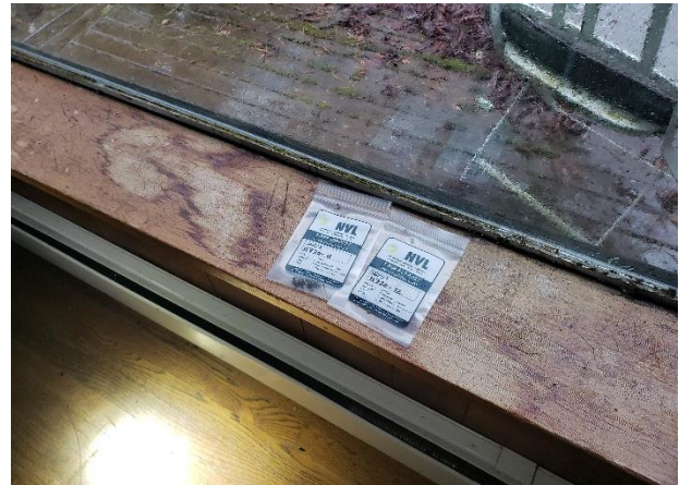
Photo #2: Samples 11720-11/11QA & 12: White interior window glazing (on 9'x11' metal frame window.) (4% Chrysotile) Location: Building 8 Living Room Interior
