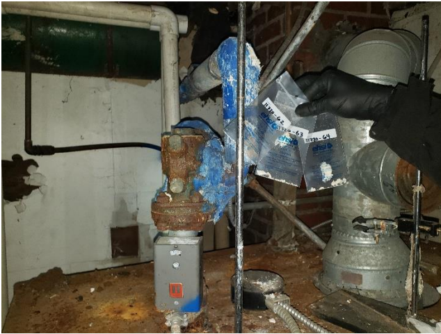
Photo #9: Samples 11720-62,63 & 64: Blue and white mudded elbows (on 4" OD metal boiler piping.) (12% Chrysotile, 5% Amosite) Location: Building 7 Garage Area
