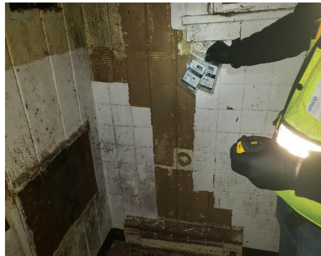
Photo #8: Samples 11720-50 & 51: 4"x4" White ceramic tile on gray grout on brown mastic (on wood paneling.) (4% Chrysotile) Location: Building 9 Bathroom
