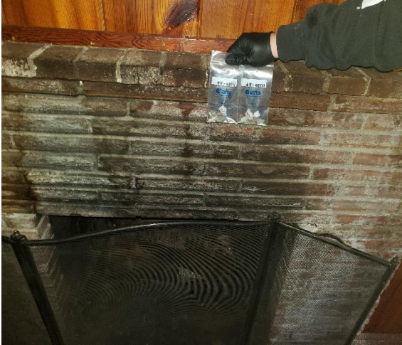
Photo #13: Samples 11720-76 & 77: Red external fireplace brick and gray internal fireplace brick on ACM mortar. (4% Chrysotile) Location: Building 6 Living Room
