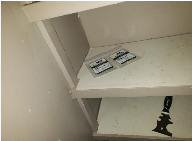
Photo #1: Samples 11720-05/05QA & 06: Beige joint compound (on GWB.) (3% Chrysotile) Location: Building 8 Kitchen
