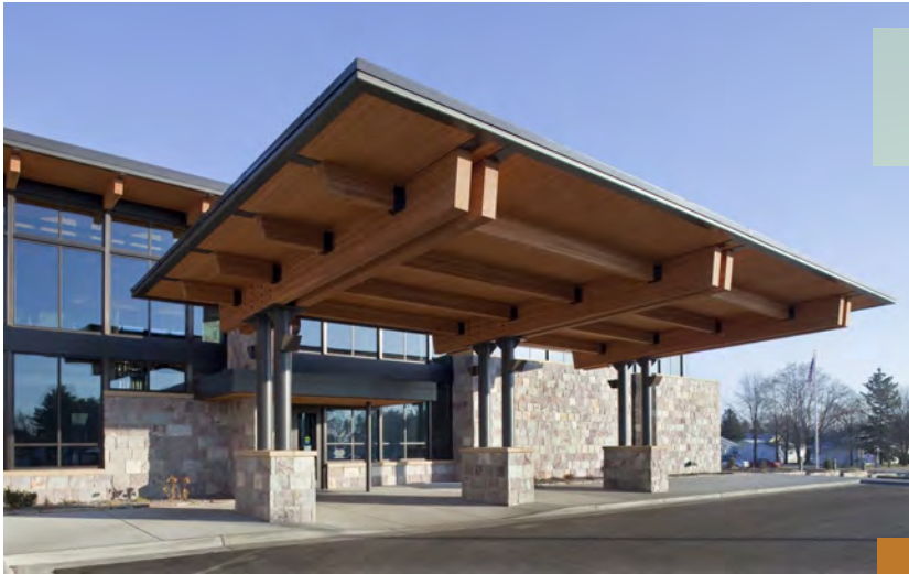
Mass Timber/GLED Laminated Timber Beams, HGA Architecture
