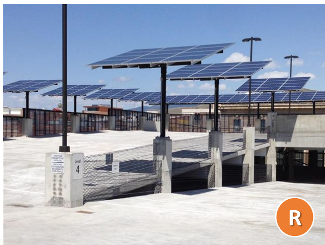
Photo voltaic solar panels that also provide sheltering/weather protection on the roof deck of a parking structure.
