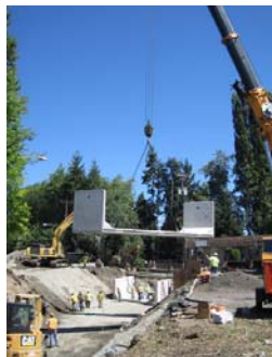
Crane placing precast concrete culvert section – SR 522 (7/10/15)
