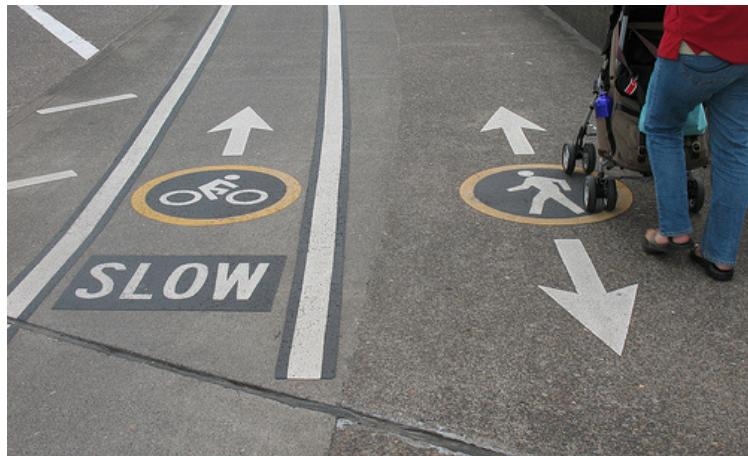
Figure 26: Shared use path pavement markings.
