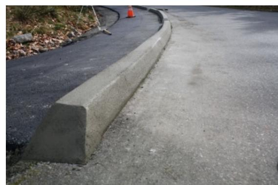
Figure 17: Pedestrian path with an extruded curb.
