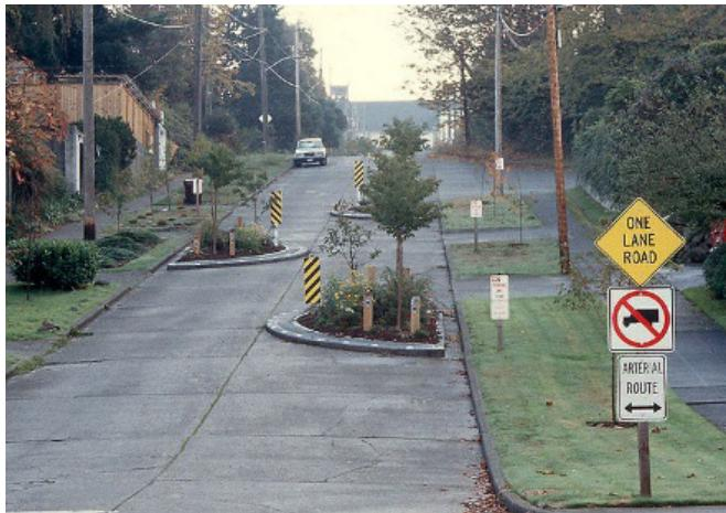
Figure 23: Example of a chicane. Source: Richard Drdul
