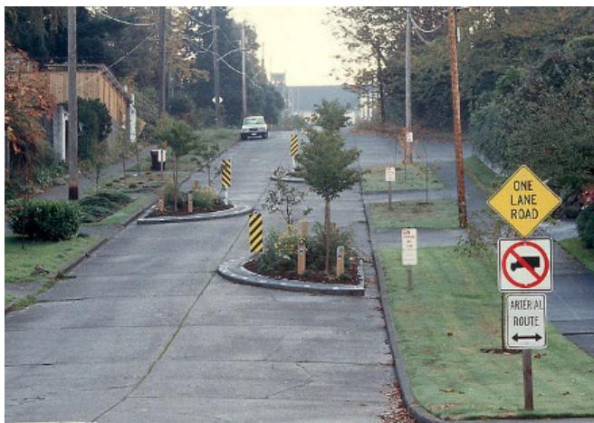
Figure 14: Example of a chicane. Source: Richard Drdul
