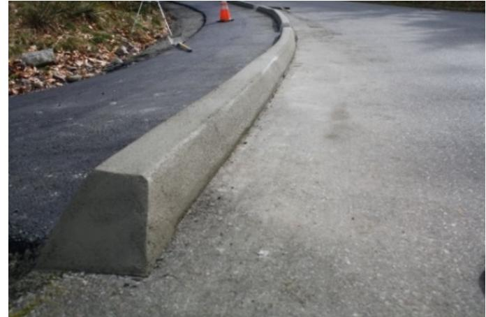
Figure 38: Pedestrian path with an extruded curb.
