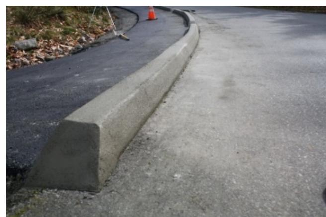
Figure 11: Pedestrian path with an extruded curb.
