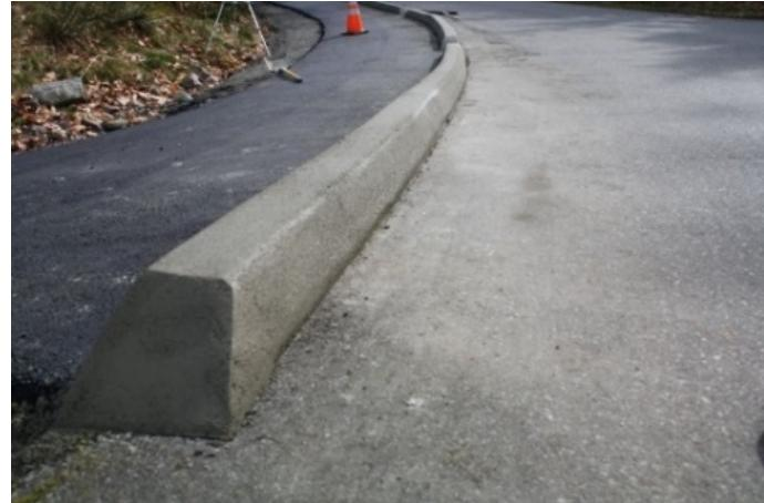
Figure 20: Pedestrian path with an extruded curb.
