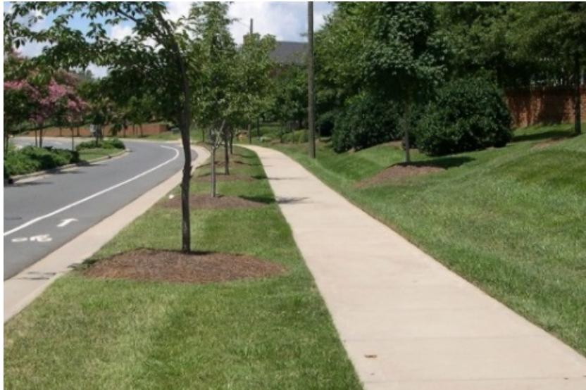
Figure 4: Sidewalk with landscaping buffer. Source: [threepullpa.com](http://threepullpa.com)
