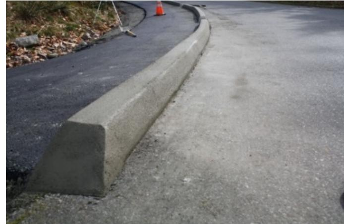
Figure 34: Pedestrian path with an extruded curb.
